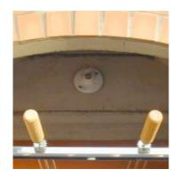
A light fixture can be easily added inside the BBQ. You must use a low profile, **surface mounted** metal electrical box, a ceramic fixture, fire proof wire and a 25 to 40 watt appliance light bulb.
